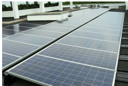
Figure 4.17: Silicio Policristalino
