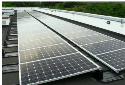
Figure 4.16: Silicio Monocristalino
